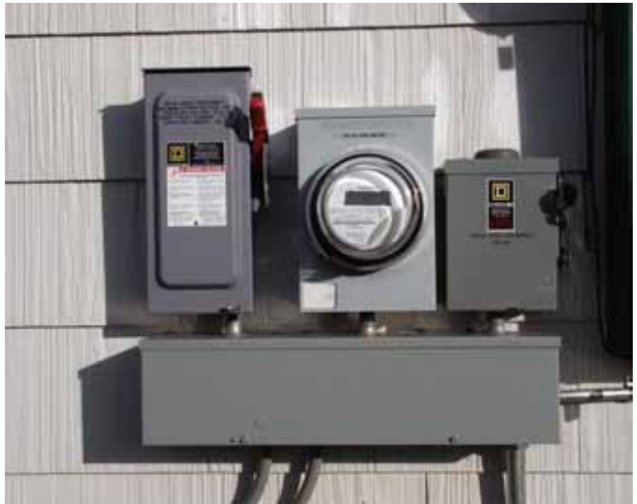
Solar array disconnect, system AC kilowatt-hour meter, and inverter disconnect mounted over a weatherproof wiring enclosure.
