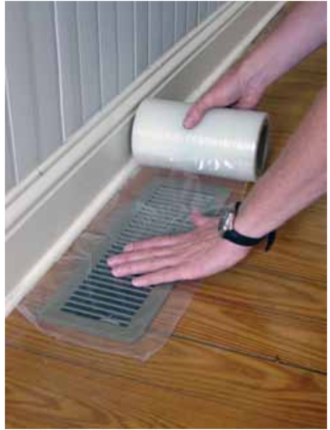
Sealing the registers in preparation for the duct pressure test.
