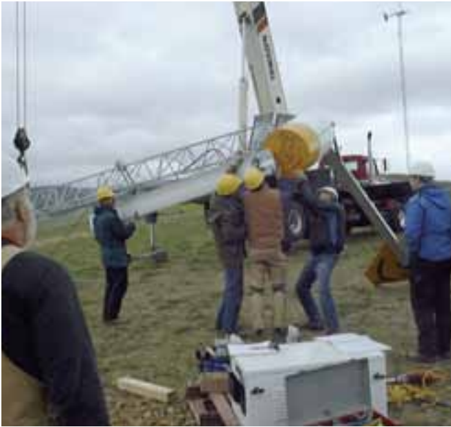
The crew installs the blades on the second Bergey Excel at the Nichols ranch.
