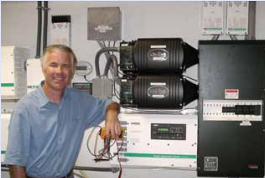
Author and system installer John McNicholas with the first stacked Xantrex/OutBack inverter system made possible by the MIG2 migration board.
