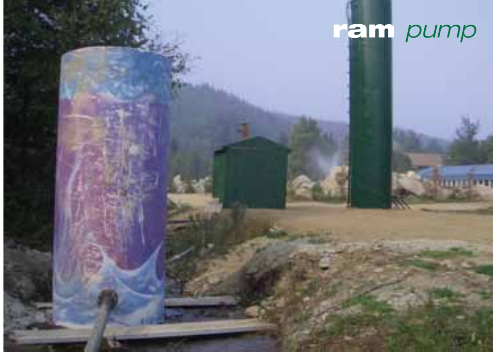
The supply tank situated in the creek, with the geothermal well house and storage tank in the background.
