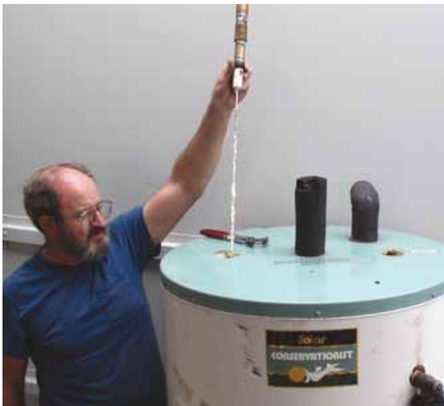
Don Keefe of AAA Solar lifts out the remains of a used-up anode rod.
