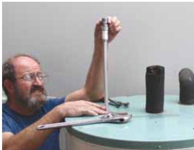
Installing a new rod in the tank.
