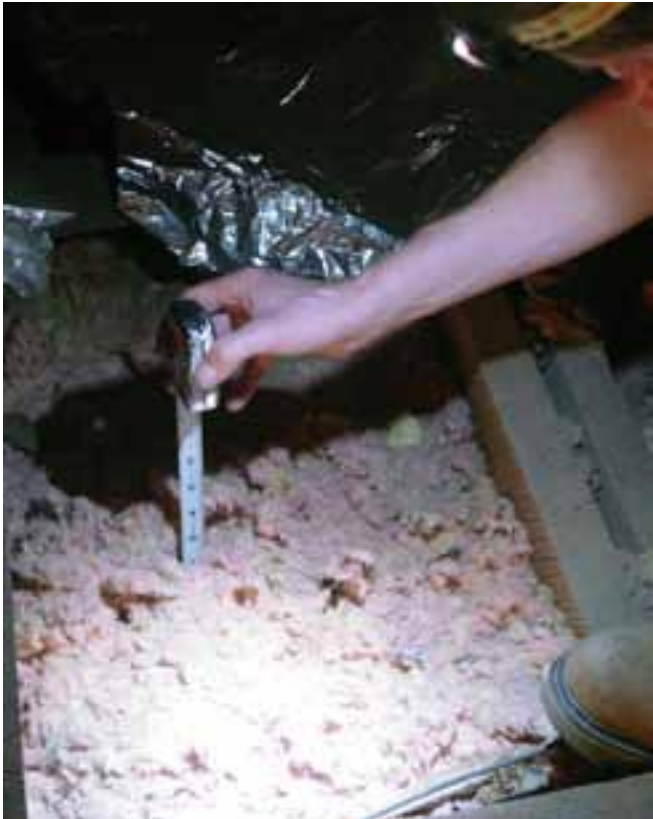
Checking the attic insulation levels.
