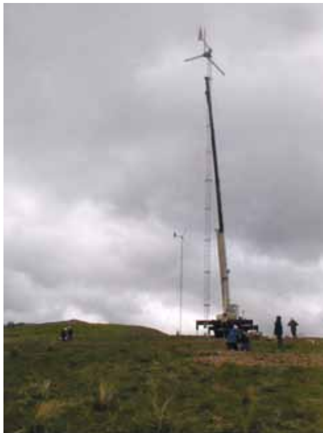
A crane lifts the second Bergey Excel wind turbine on a 100-foot (30 m), guyed, lattice tower.
