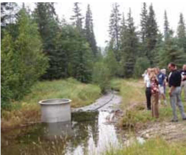
Gwen at the dam site, with the partially buried stainless steel inlet.
