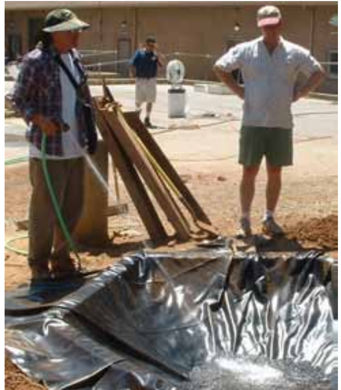
The liner is laid into the hole dug for the fountain basin and across the fountain curb. Water is added before the liner is tacked to the wooden curb to allow for an unstressed fitting.
