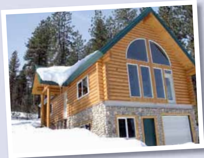
With logs having an insulation value of only R-1 per inch of wood, adding SIPs to the roofing system of this home makes the whole building more efficient.
