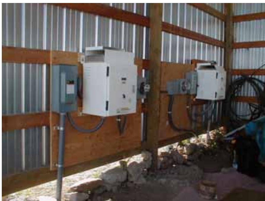
Dual GridTek inverters convert the three-phase wild AC output of the Bergey Excel wind turbines to grid-synchronous AC.
