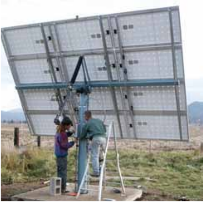
Joe and Daniel put the finishing touches on the tracked PV array.
